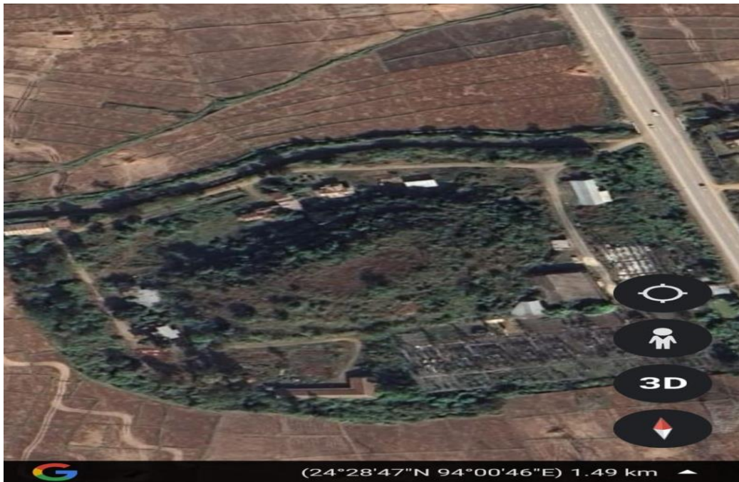
Satellite Image of 132/33 KV Kakching Power Sub-Station at Kakching District
